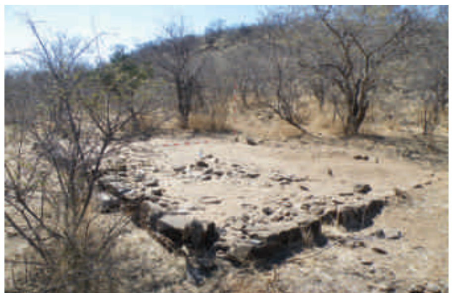
Figure 13 Rectangular building with some foundations at KWH1
