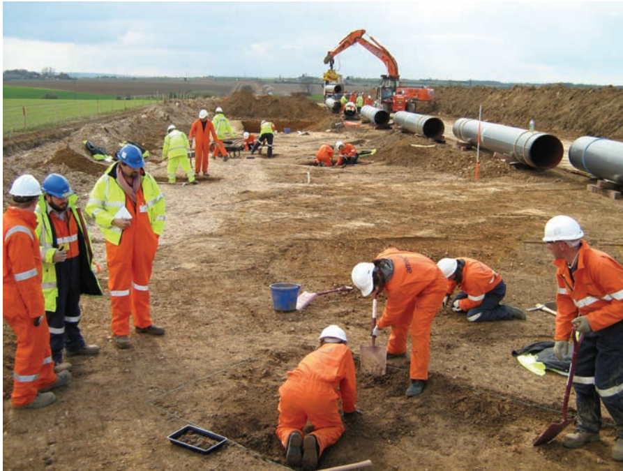
Figure 2 Excavations along the Grain to Shorne gas pipeline in Kent
