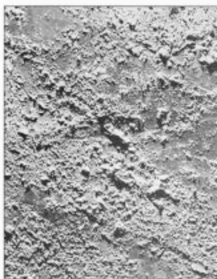
Figure 5 Detail of salt damage to part of a thirteenth-century wall painting on the south wall of the sacristy of Cleve Abbey, Somerset, 1997.
