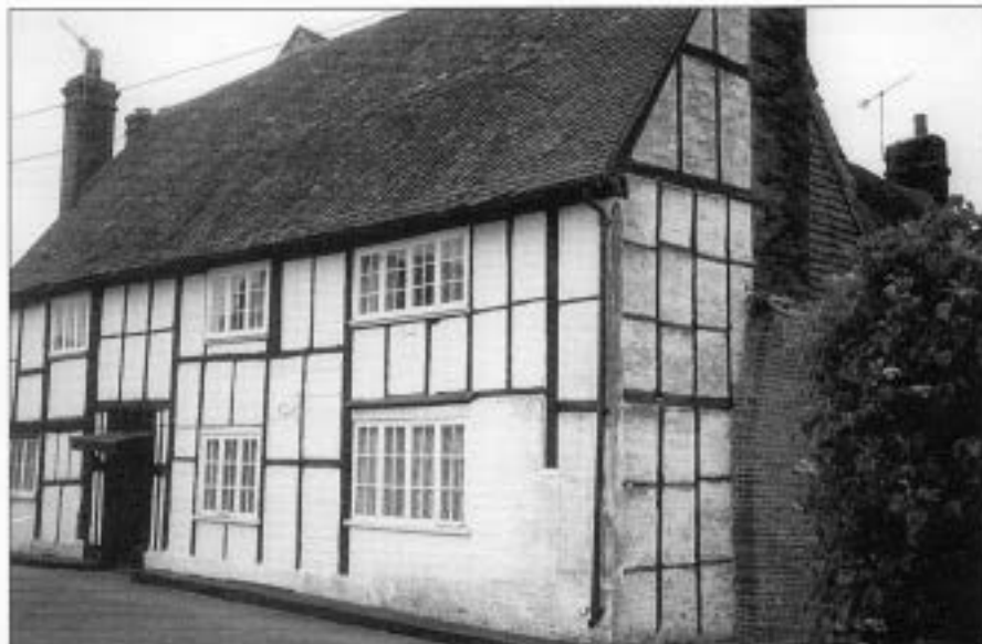
Figure 5 View of the east facade of the farmhouse at Home Farm, Newdigate, Surrey, built of timbers felled in the period 1574–1603.
