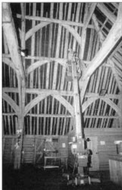
Figure 4 Internal view of Priory Barn, Little Wymondley, Hertfordshire, showing the author taking samples for dendrochronological study.
